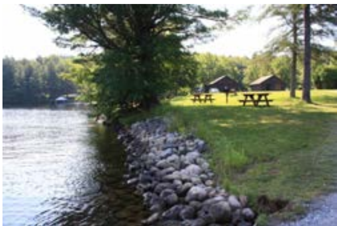
Shoreline Protection at Day Use Area
