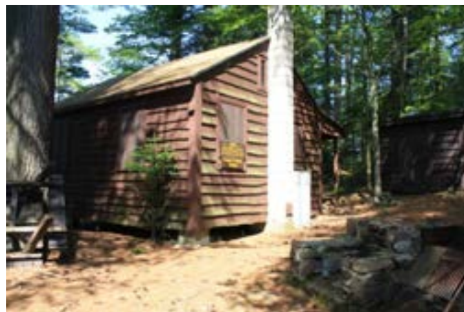
Alger Island Caretaker's Cabin
