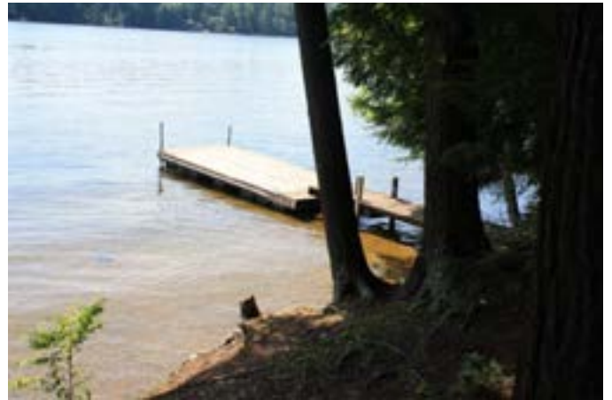
Alger Island Day Use Dock
