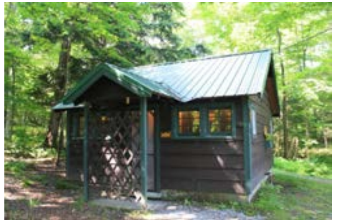
Day Use Area Comfort Station
