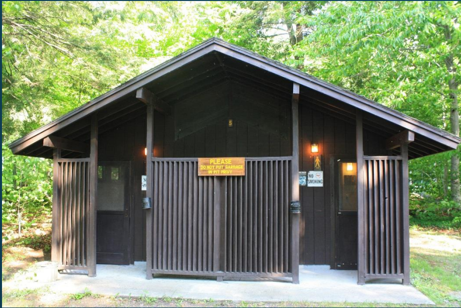
Little Sand Point Comfort Station #1
