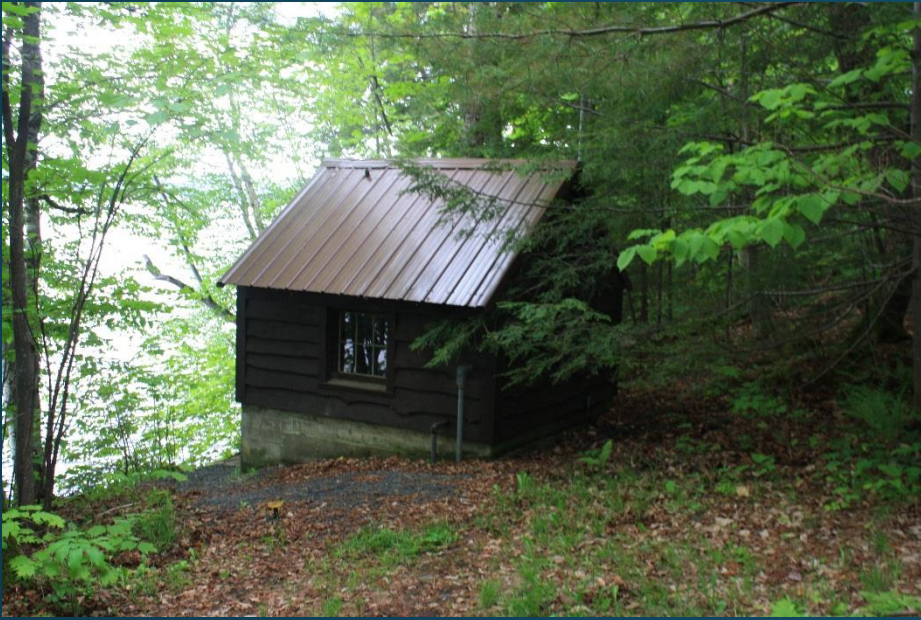
Little Sand Point Water Pump Station
