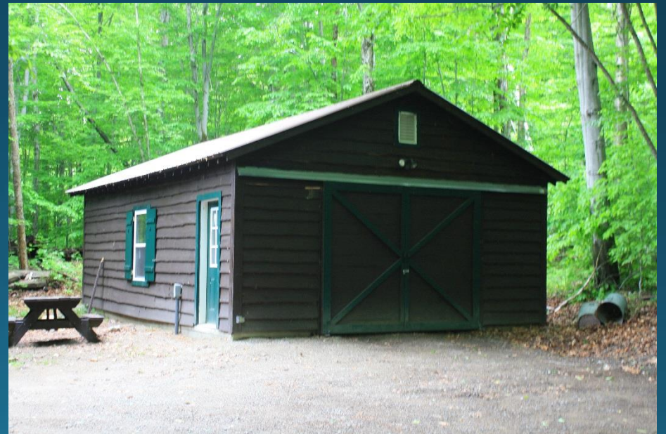
Little Sand Point Wood Storage Building
