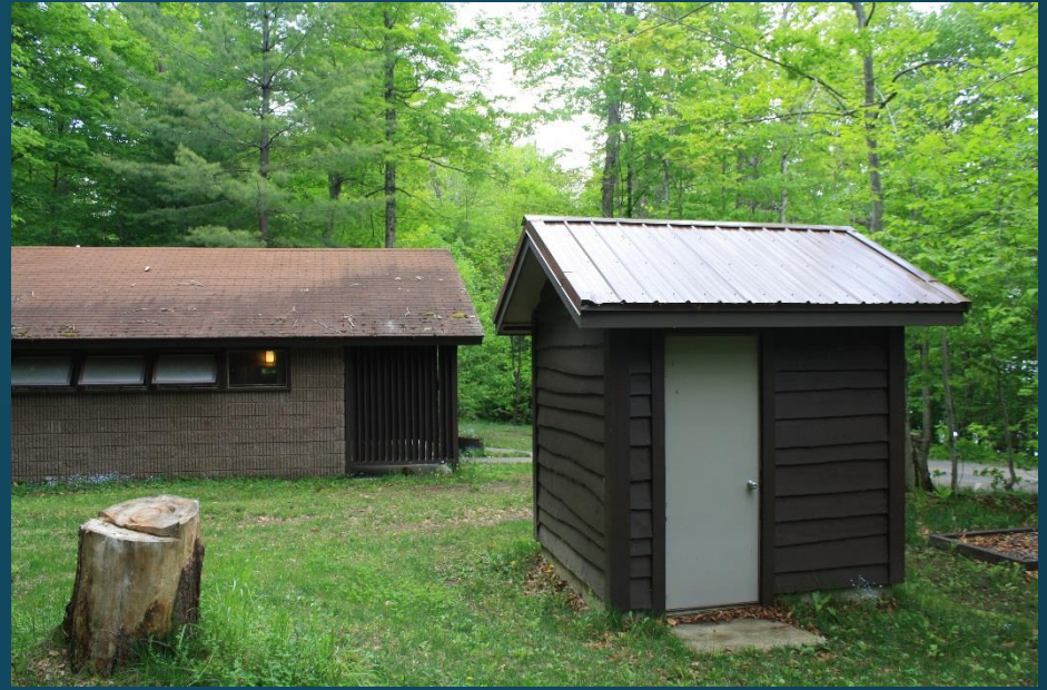
Little Sand Point Sewage Lift Station
