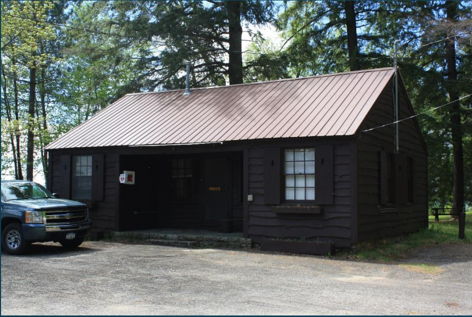
Poplar Point Caretaker Cabin
