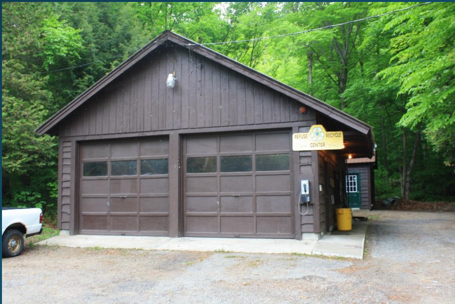
Little Sand Point Garage
