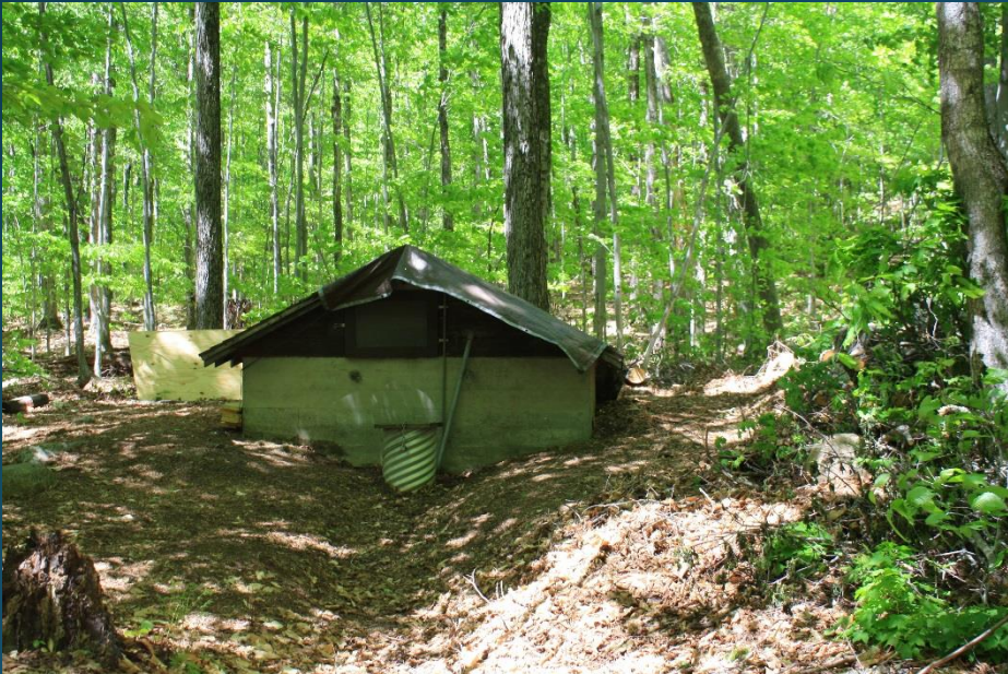
Poplar Point Reservoir
