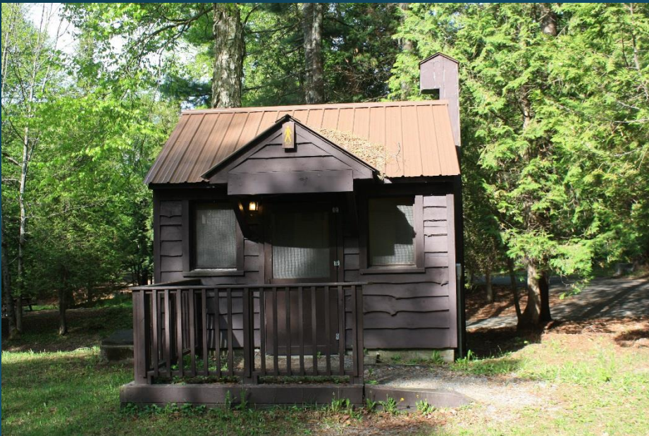
Point Comfort Comfort Station #3
