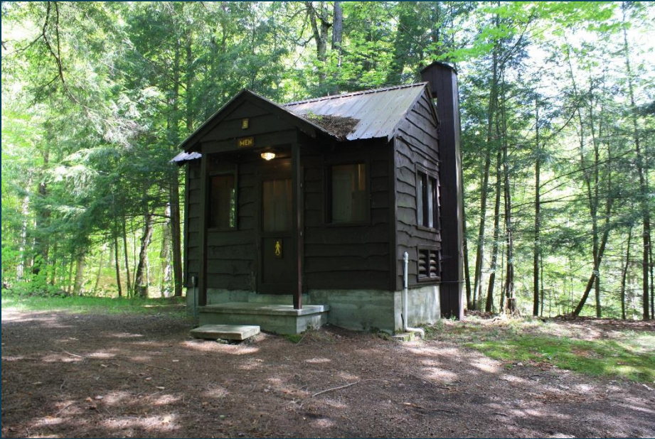
Point Comfort Comfort Station #1
