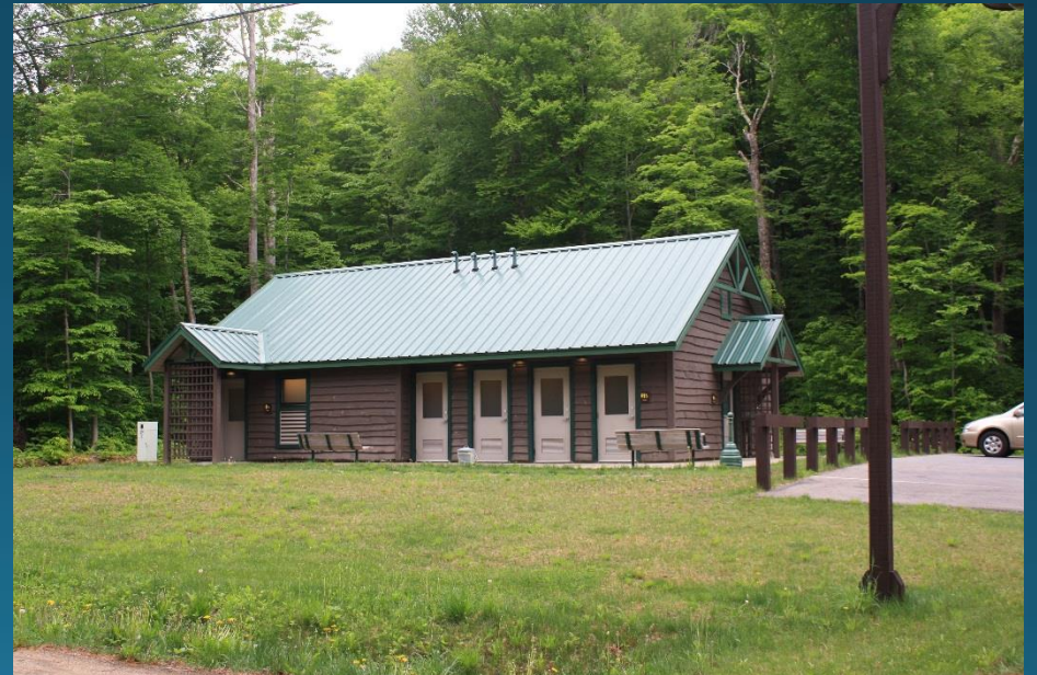
Little Sand Point Shower Building
