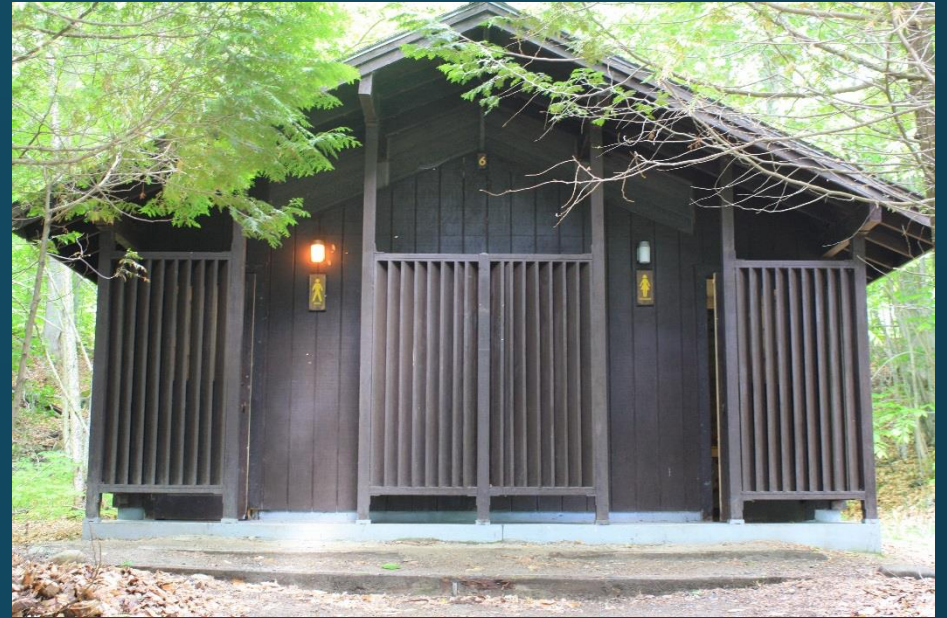
Little Sand Point Comfort Station #2
