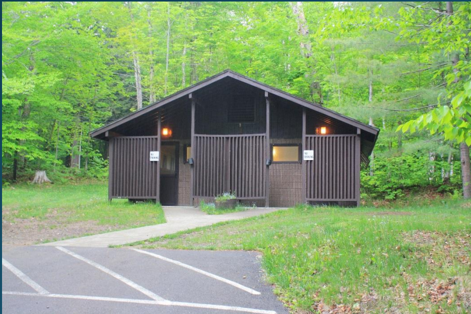
Little Sand Point Comfort Station #3
