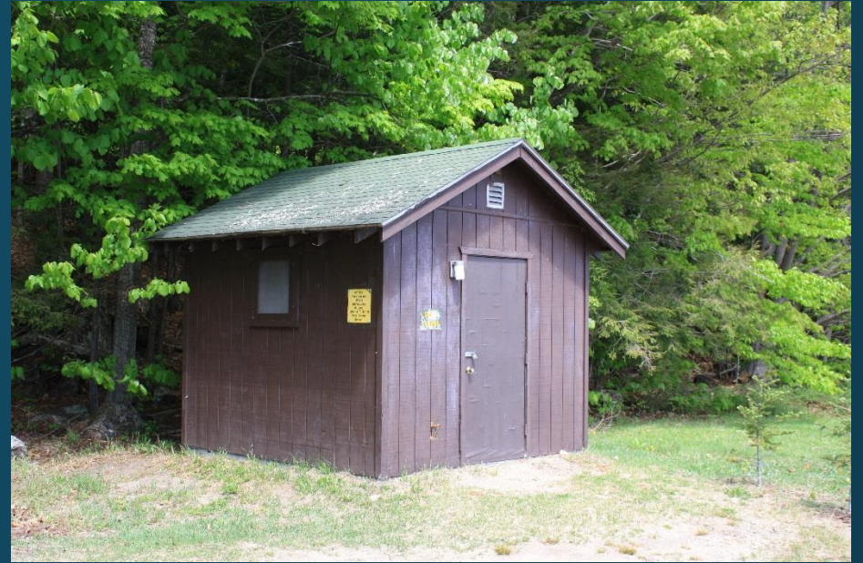
Poplar Point Pump House
