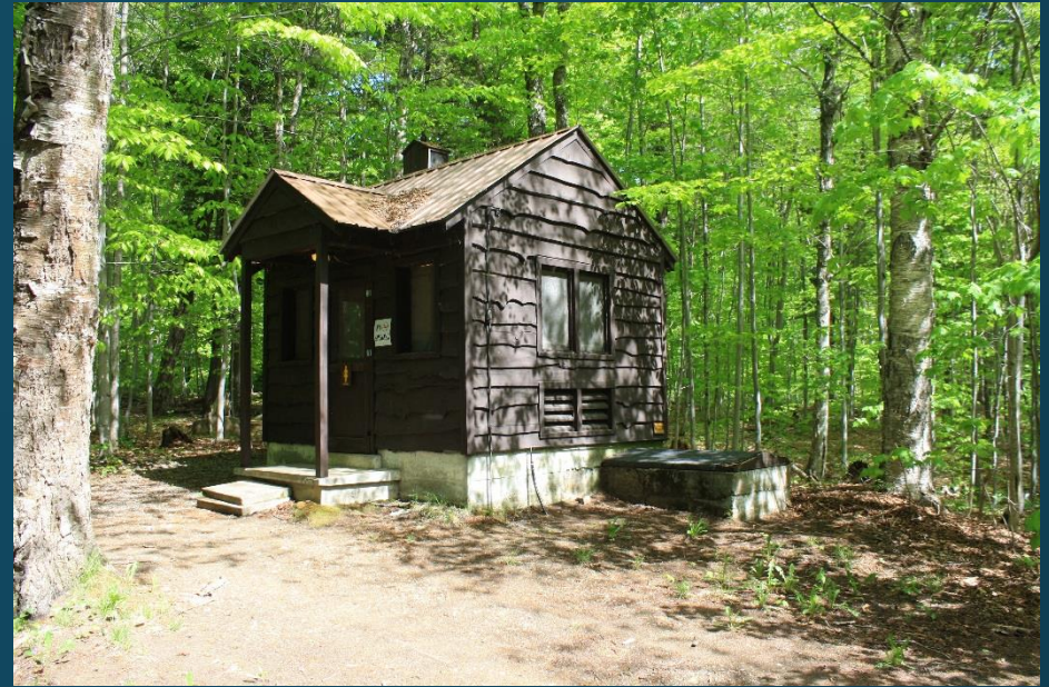
Point Comfort Comfort Station #2
