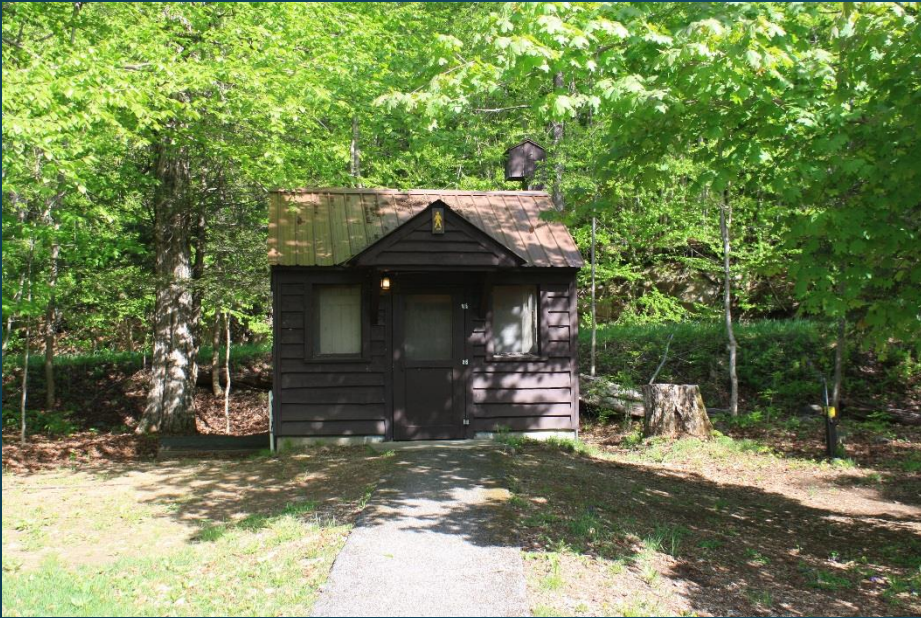
Point Comfort Comfort Station #5
