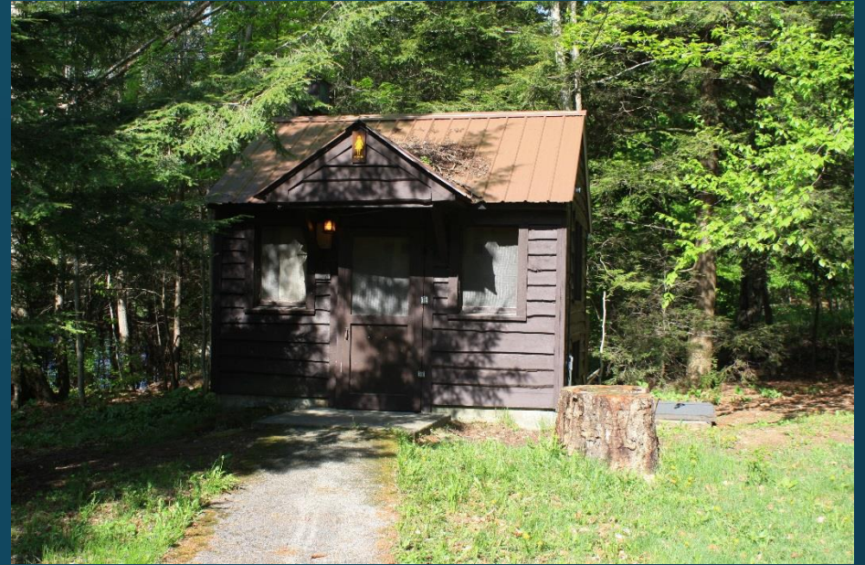
Point Comfort Comfort Station #6
