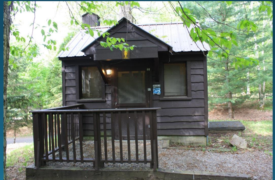
Point Comfort Comfort Station #4
