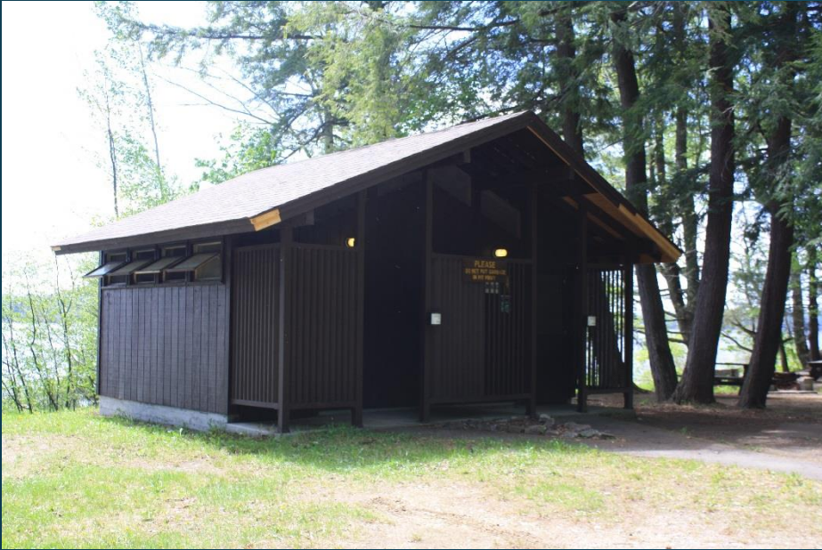
Poplar Point Comfort Station
