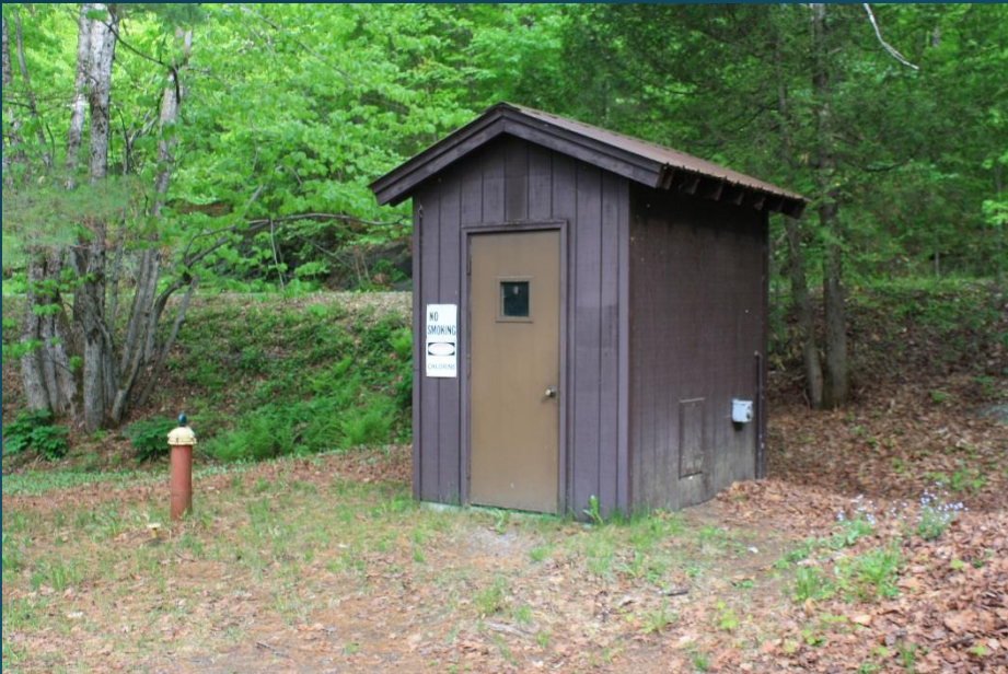
Point Comfort Pump House
