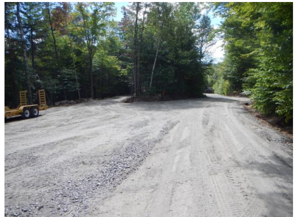
Lower Parking Lot on Gulf Brook Road
