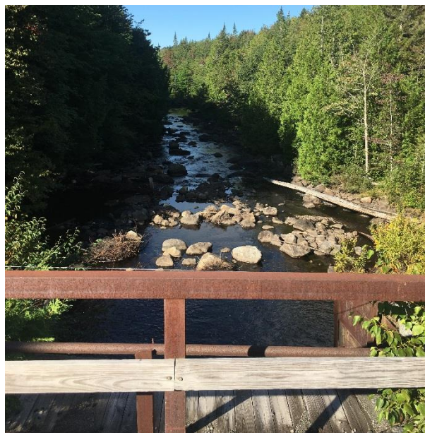
LaBier Flow Bridge over the Boreas River
