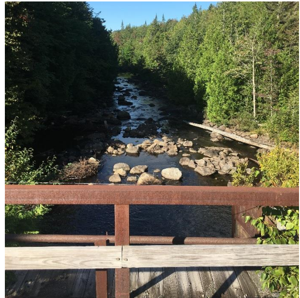
LaBier Flow Bridge over the Boreas River
