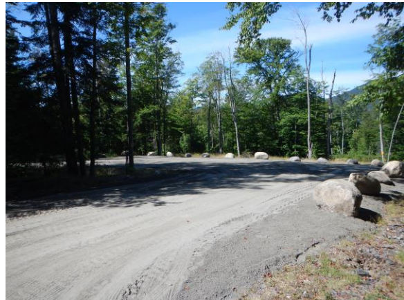
Upper Elk Lake Road Parking Area, 2016
