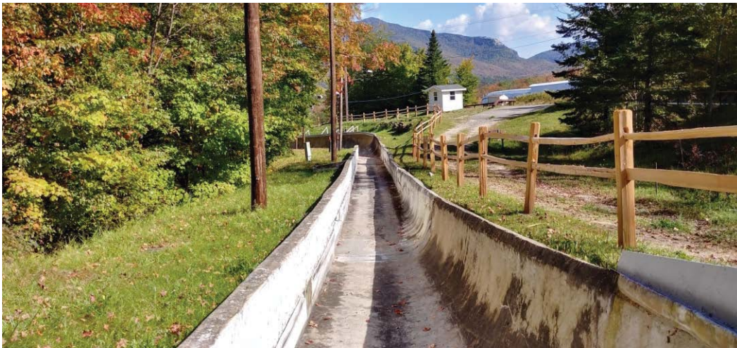
Exit Little S (Photo #14)
