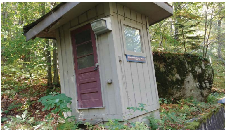
Communication Shack (Photo #3)
