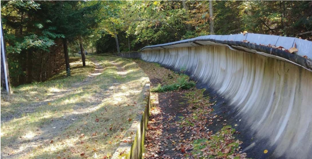
Uphill Curve 5 (Photo #1)
