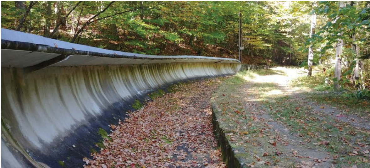
Uphill Curve 7 (Photo #5)
