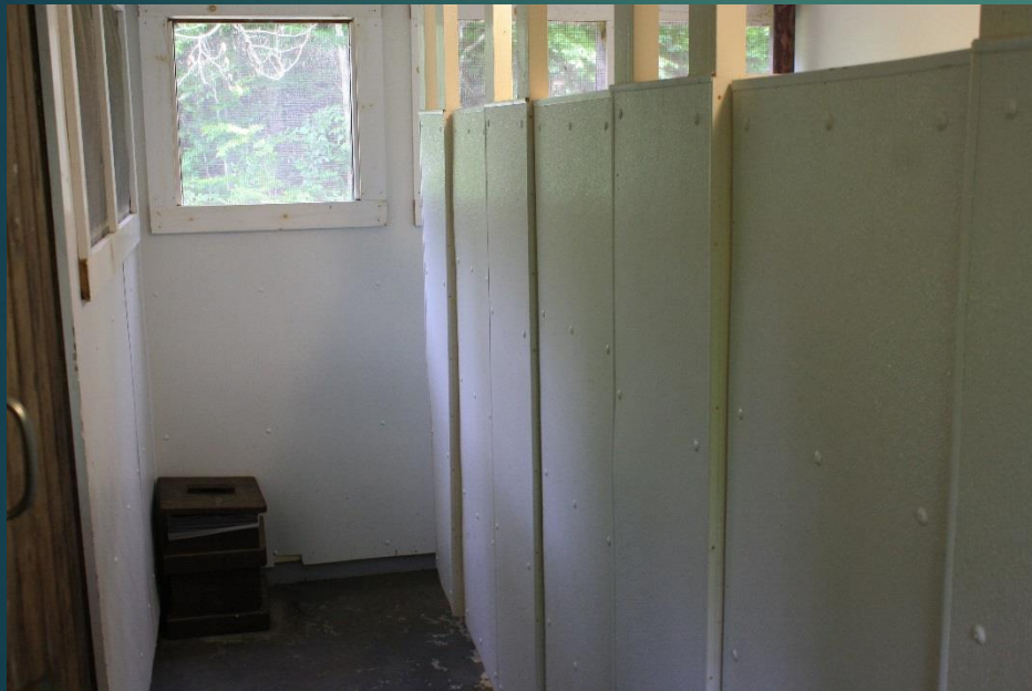
Interior of Toilet Buildings
