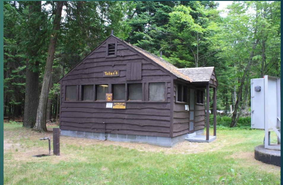
Toilet Building #4 - Day Use Area
