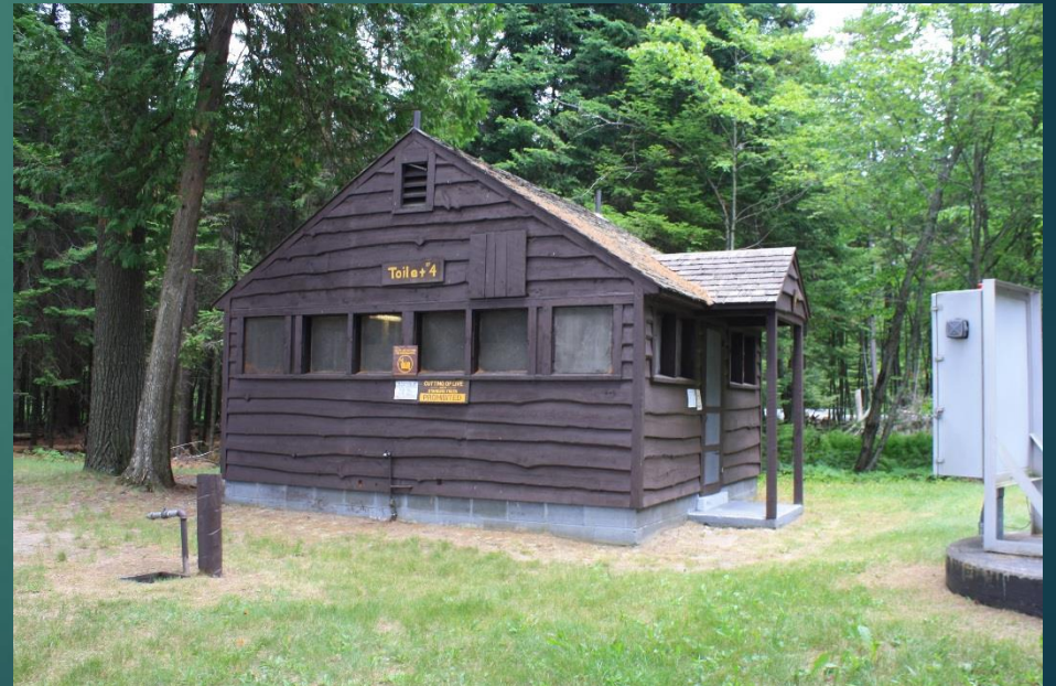
Toilet Building #4 - Day Use Area
