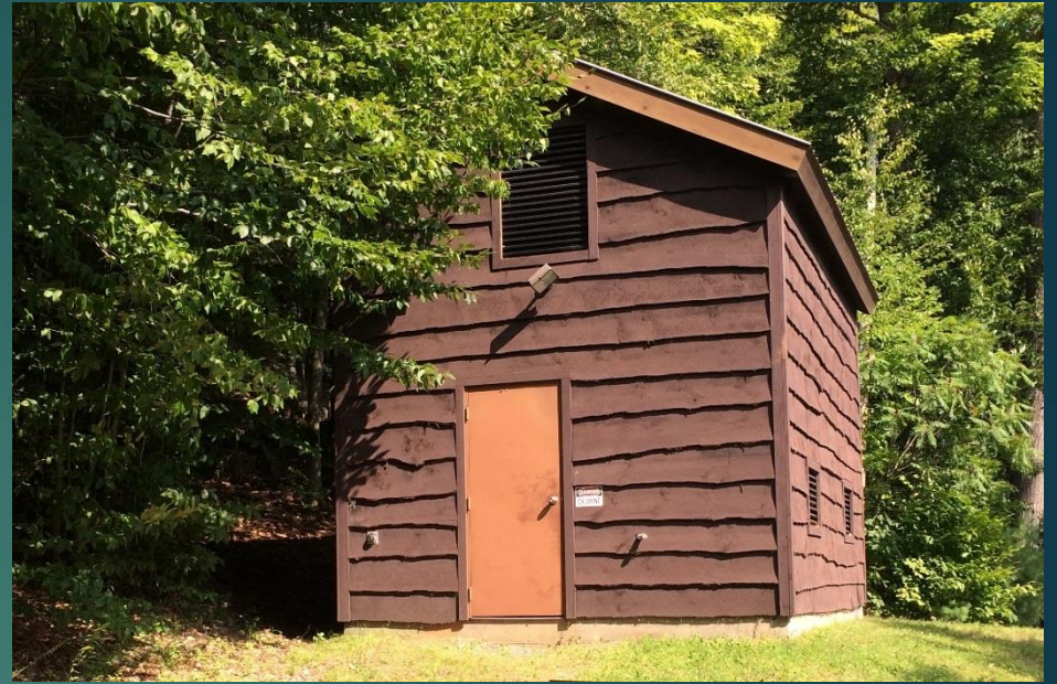
Chlorination & Reservoir Bldg
