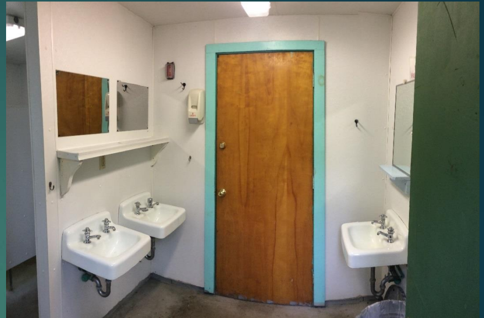
Shower Building Interior
