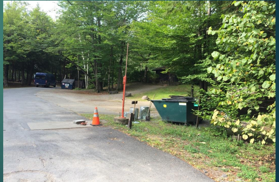
Trailer Dump Station
