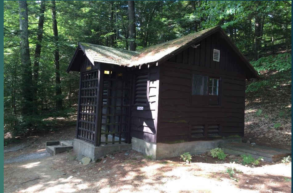
Beach Road Comfort Station (11)
