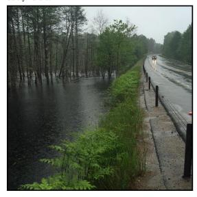
impound water which may flood or wash out roads. Upstream and downstream impoundments must be monitored and removed as necessary to prevent washouts of culverts and embankments. Damage also occurs when a roadbed becomes saturated with water and settles. The overall stability of the road decreases as the pavement becomes stressed and potholes form. Nuisance
