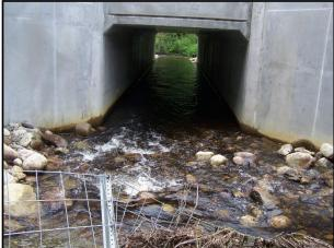
Measures that support wildlife also support transportation systems. For instance, larger structure openings (with upland areas) can facilitate bridge maintenance activities by providing a dry work area adjacent to the water feature. Larger openings also can accommodate greater flow passage during storm events, with an understanding that a hydraulic analysis is needed to be sure downstream flooding is not increased.
