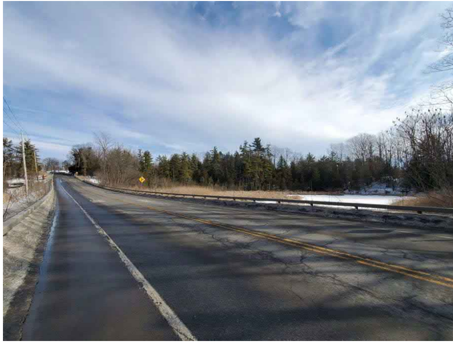
Photo 1: View of evergreen vegetative buffer on southern end of the Project Site from 9N/22, facing north.
