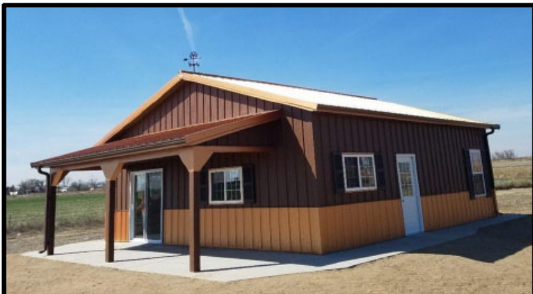
Maintenance/ mechanical building – 900 sq ft / 32 ft max height
