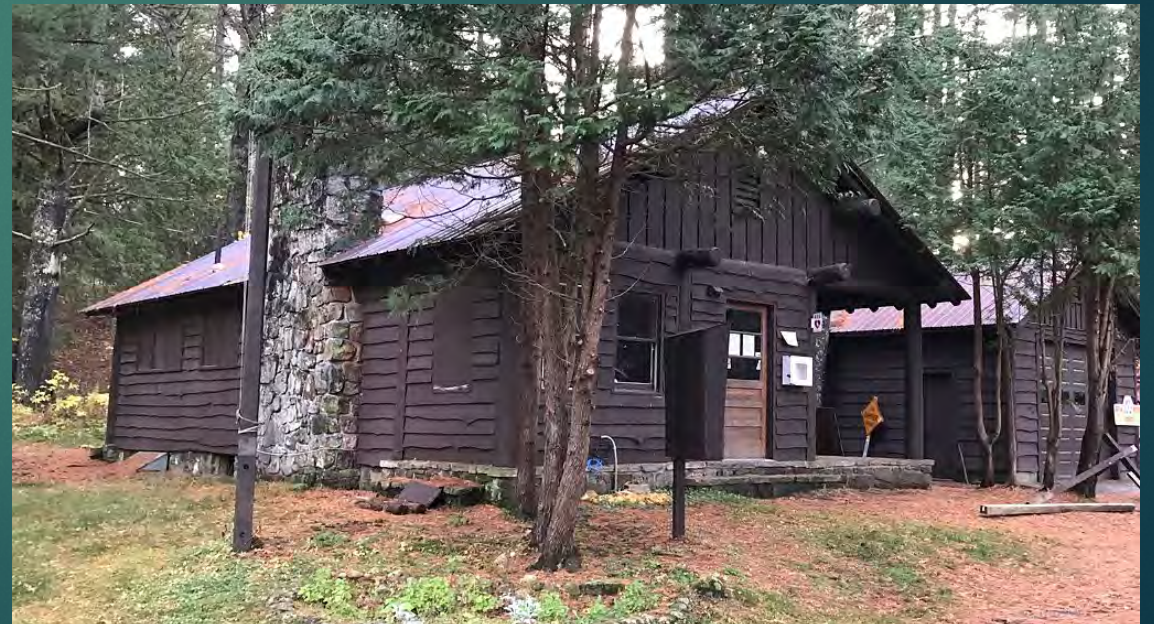
Caretaker Cabin and Office.
