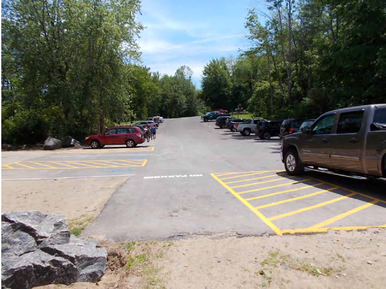
Figure 8. Photo of existing beach parking area.
