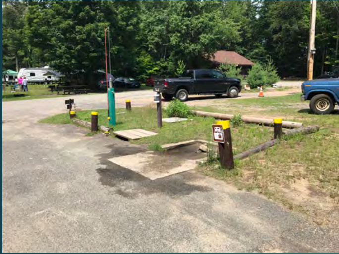
Trailer Dumping Station
