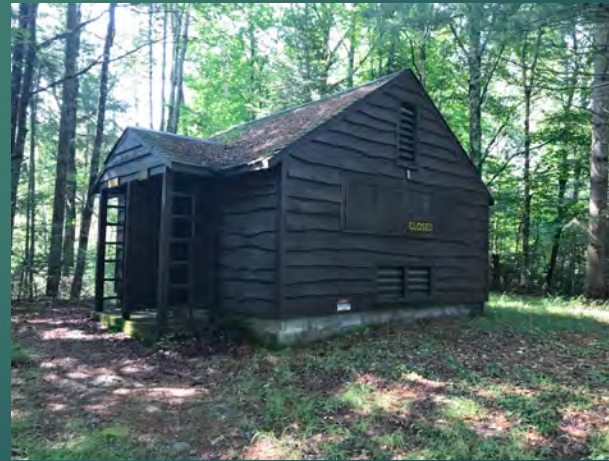
Vault Toilet Building
