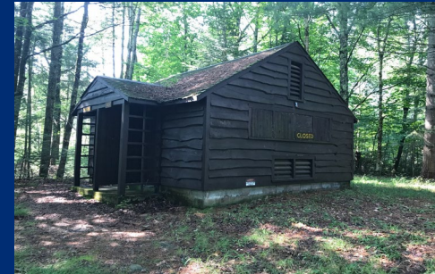
Vault Toilet Building #7
