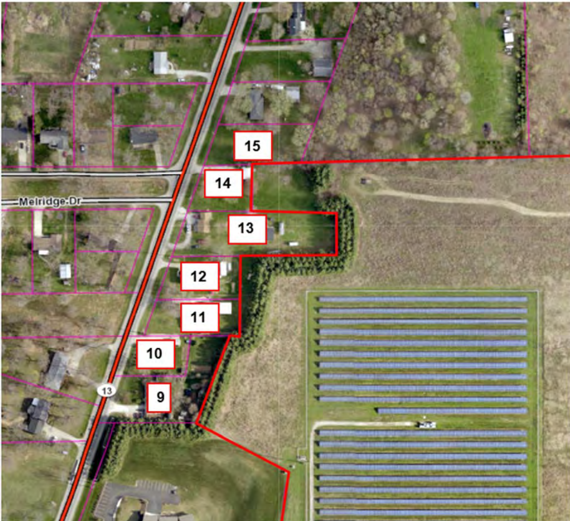
Solar Farm 6 Adjoining Properties
