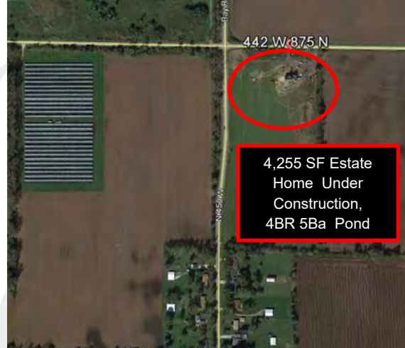
Portage Solar Farm (Solar Farm 2) October 2016
