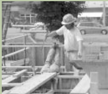
Left: (from left) Joe Rota and Frank Mezzano pictured with 2003 Earth Day Awardees, Lloyd Moore, George Canon, Dick Lefebvre, and Chris Westbrook. Chairman Frenette is pictured far right; Right: Construction workers prepare foundation for new conference room at Ray Brook headquarters.
