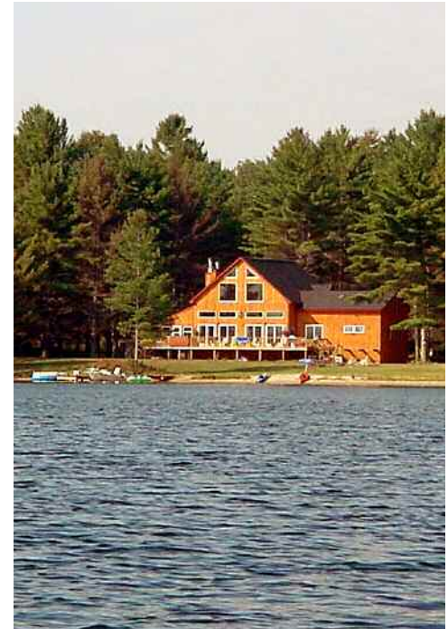
The owners of this house on Lake Clear were required to remove an illegal deck, plant significant vegetation and pay a civil penalty to resolve violations of the APA Act.
