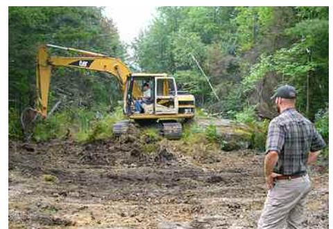
Enforcement Officer John Burth oversees the removal of fill that was illegally placed in a regulated wetland.
