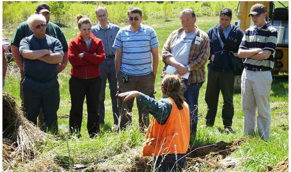
Project Analyst Lawrence Phillips, standing in trench, and Environmental Engineer Greg Bendell, second from right, conduct a deep hole test pit training workshop for local government officials and contractors.
