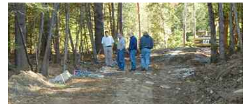
Agency staff inspects an access road.
