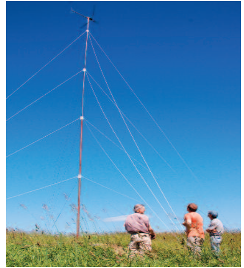
Leigh Walrath (center) conducts a site visit for a wind turbine project in the Town of Essex.
