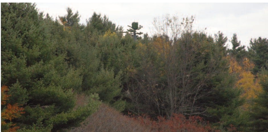
Centered above is a permitted simulated white pine cellular tower recently constructed in the vicinity of Northway exit 27 in the Town of Schroon.
