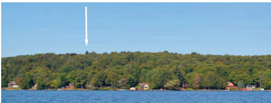
The above 105 foot tall cell tower is located in the Town of Clifton, St. Lawrence County. The top portion was fabricated as a simulated pine tree to help blend the tower into the landscape. Click for Towers Policy
