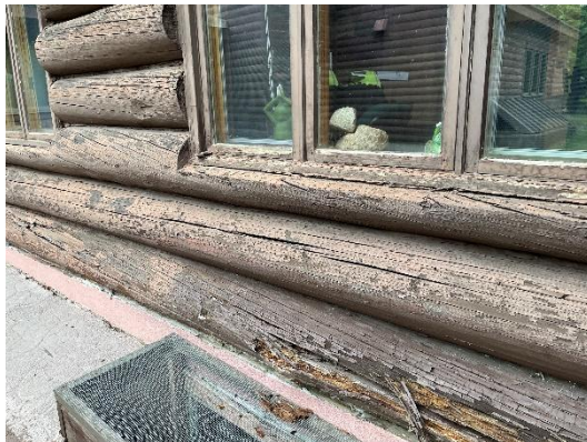
Photo 9 – Deteriorated Log
