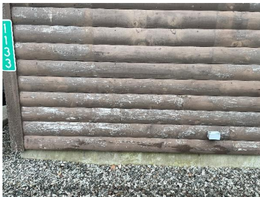
Photo 17 – Failed Paint Coating
