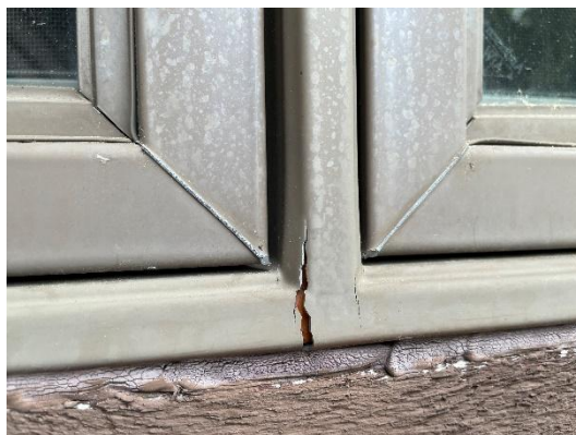
Photo 23 – Cracked Cladding
