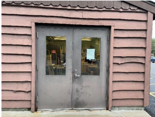
Photo 19 – Corroded Steel Frame
