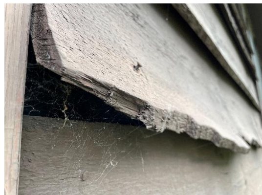
Photo 12 – 90's Siding w/ Severe Cupping
