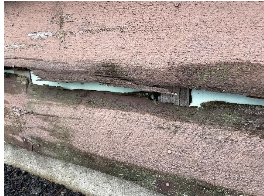
Photo 14 – 2004 Rot w/ Exposed Insulation
