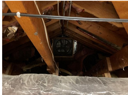
Photo 28 – Vent with Fan (Disconnected)
