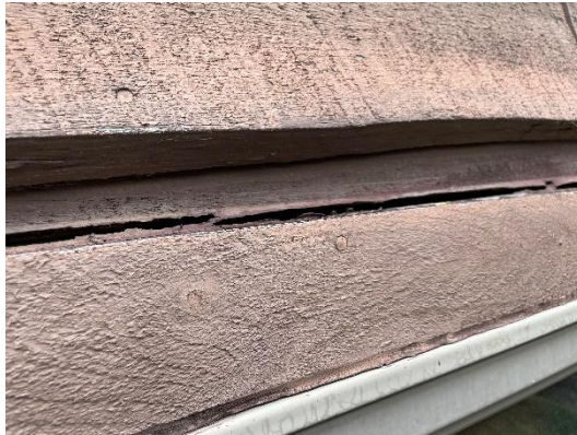
Photo 13 – Splitting Typical
