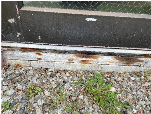
Photo 21 – Deteriorated Wood Sill
