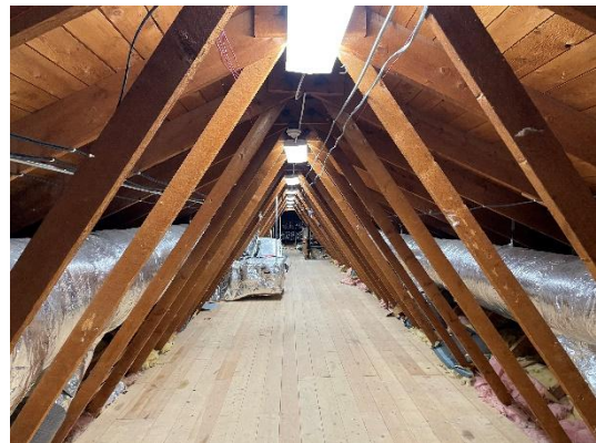
Photo 32 – Uninsulated/Vented Attic Space
