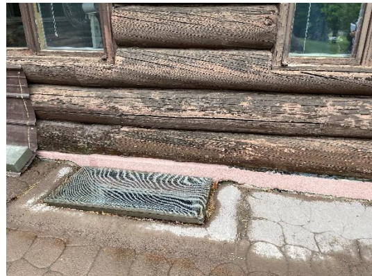
Photo 10 – Deteriorated Log
