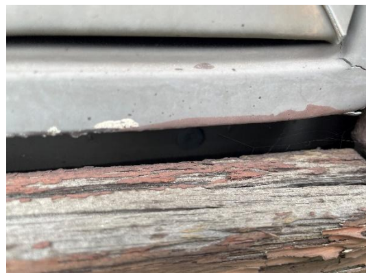
Photo 24 – No Sill Flashing or Sealant
