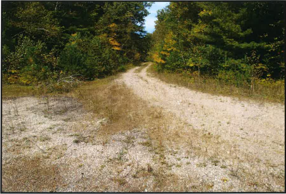
Photograph 3) View of the access road as it enters the active mined area.
