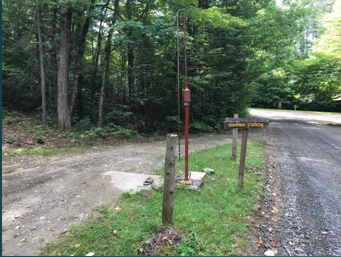
Trailer Dumping Station
